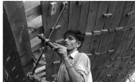
Figure 2: Fixing Wooden Wall on the Ribs of the Boat.(Source: NCMPR Depository)
